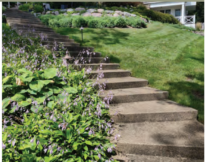
Would this beautiful walkway be safer if it had a railing?
