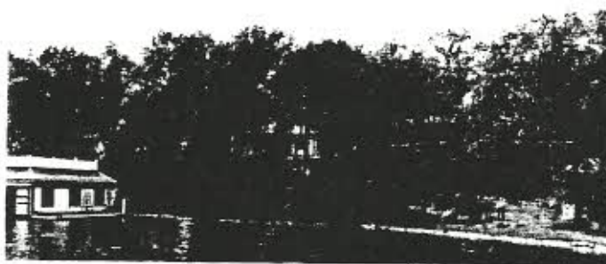
Johnston home, first house built on Lake Beulah
